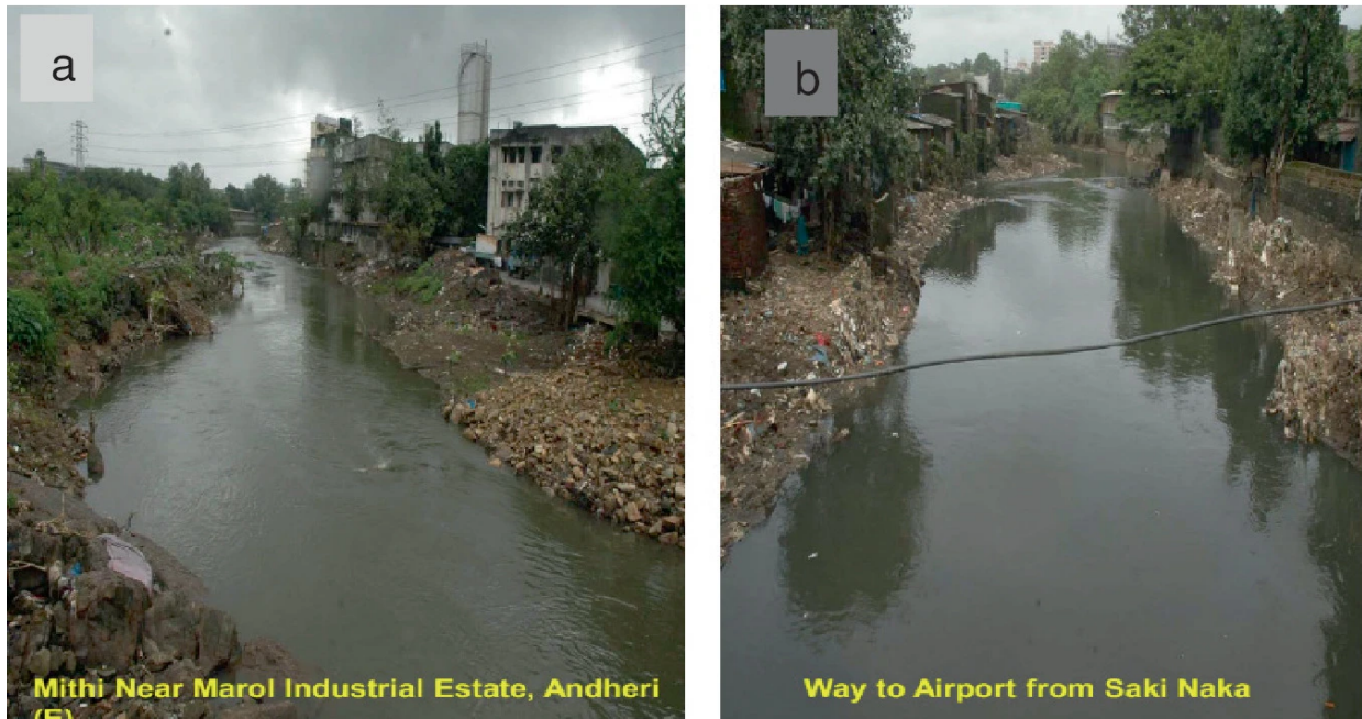
Figure 12: Pollution along the Mithi Nadi (obtained from Maharashtra Pollution Control board)
