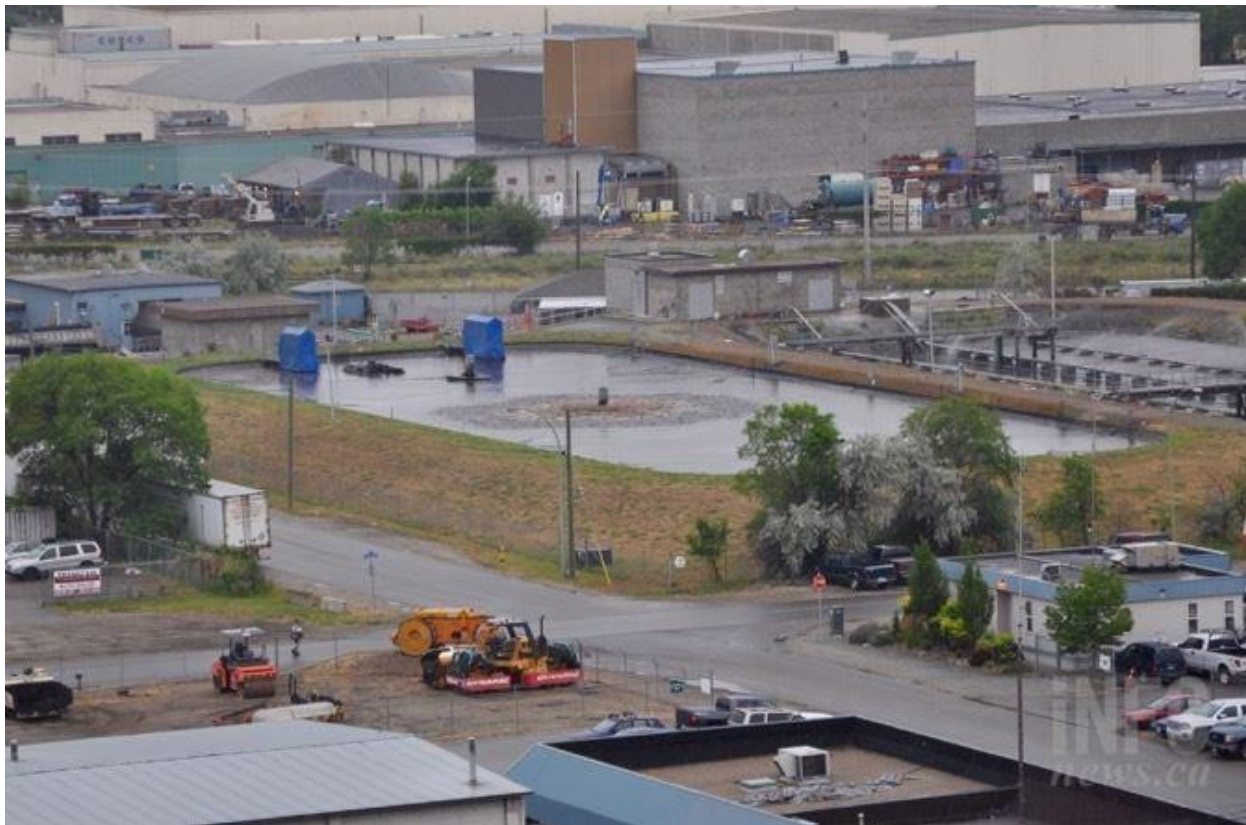
Figure 5.2.3 - Brandt's Creek Trade Waste Treatment Plant
