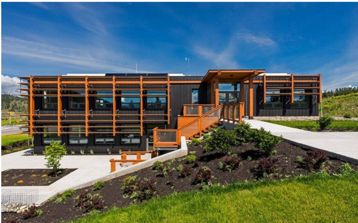
Figure 12: Energy efficient Glenmore Landfill Administration Building (Source: Naturally Wood)
