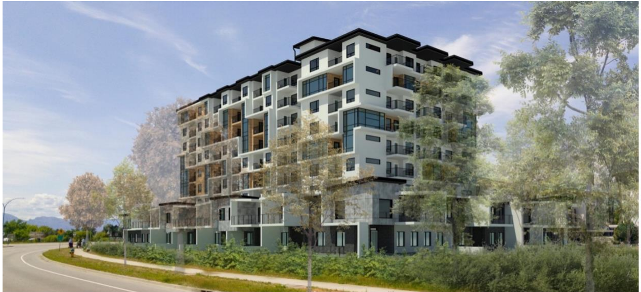
Figure 16: New energy-efficient and affordable rental housing under construction in Kelowna (Source: ROV Consulting 2020)
