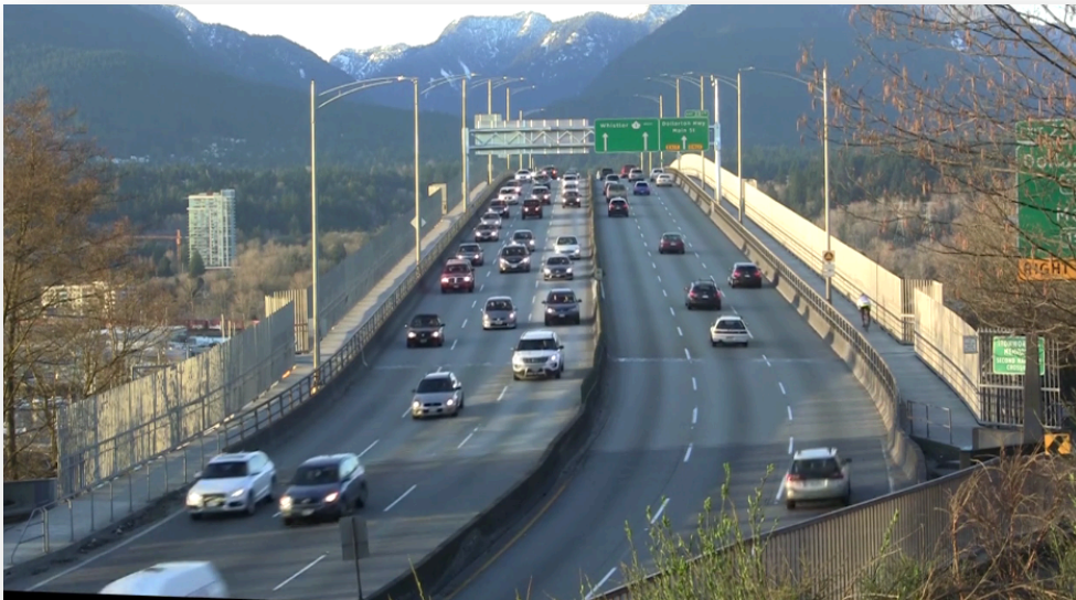
Figure 16 - Still From: Urban-Iron Workers Memorial Bridge – SLOW MEDIA Community
