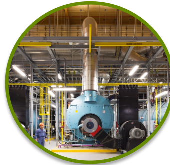
Campus Energy Centre
