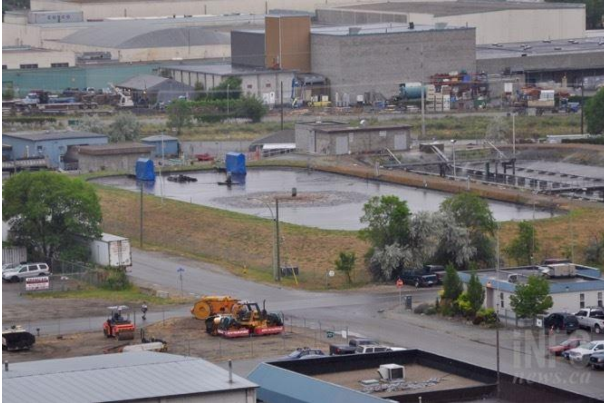
Figure: Brandt's Creek Trade Waste Treatment Plant.
